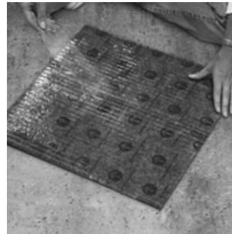
Remove peel-off backing and slide carpet tile into position on the floor.
